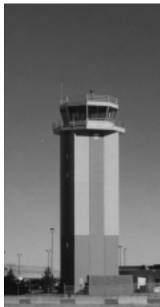
Cheyenne's New FAA contract control tower
