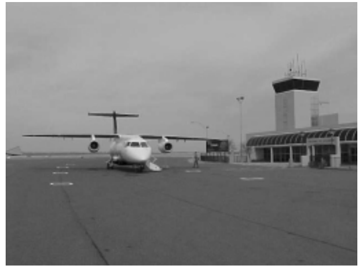
Stillwater, Okla., Celebrates New Contract Control Tower
